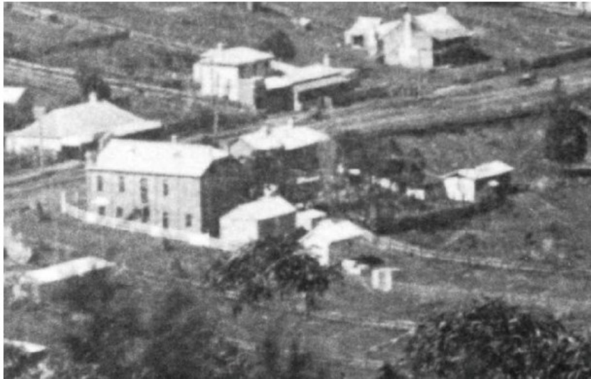
Plate 9: Photo of the School of Arts and Police Sergeants Quarters on the centre left with the subject site at right. Note: the Post Office is now two storeys. (Gosford City Council Photo Collection dated 1908)
