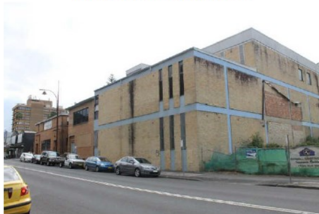
Plate 33: A view looking north on Mann Street towards the Telephone exchange and Post Office showing the Administration building in the background as seen from street level. (Source - JBA)
