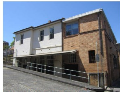
Plate 24: The building today. (JCHD DI 0420)
