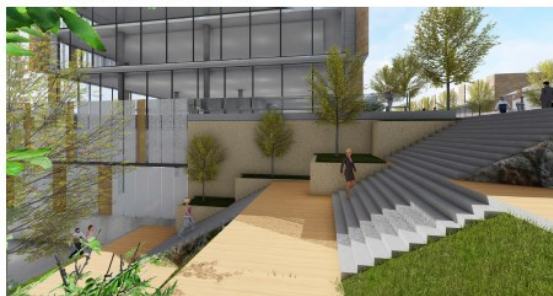
INDICATIVE VIEW FOR THE FUTURE CONNECTION
